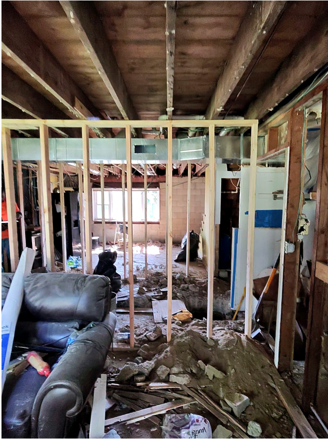
Gut renovation — framing work.
